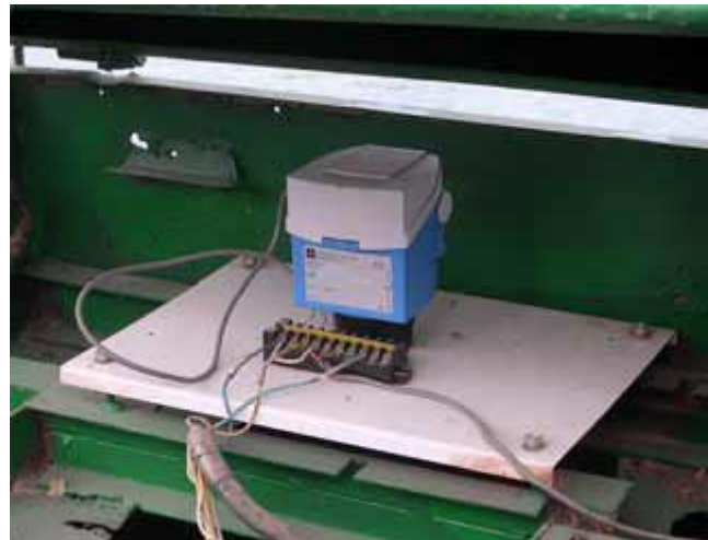
Figure 2. Installation of the water level sensor.
