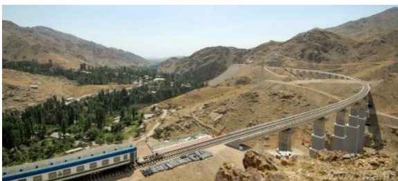
Fig. 2. Dangerous railway lines in the mountain ranges of the Republic (Angren-Pap)
